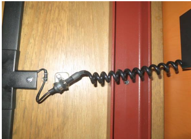
Figure 25: DC connectors mounted to a table using a clamp
