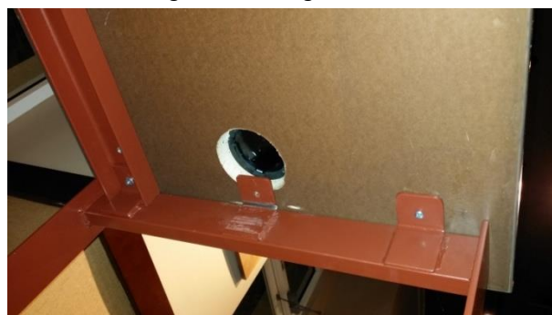
Figure 2: Drilling over a bracket
